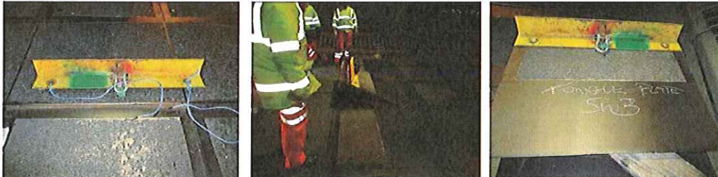
Fixing of lifting eye beam for removal of slide train
