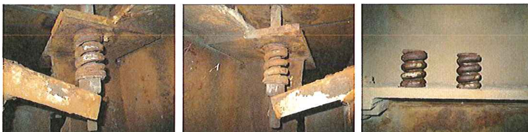
General condition of springs during pre-inspection
