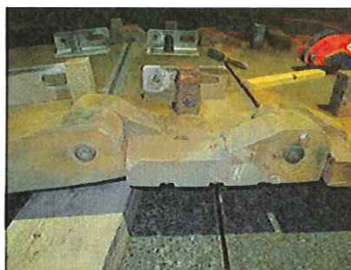
General Condition of Slide Train Pins and Bushes
