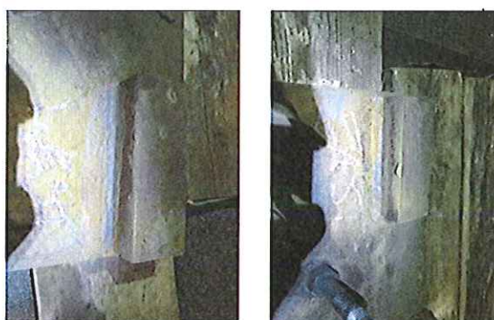
Rocker Plate End Bearing Blocks (East and West)
