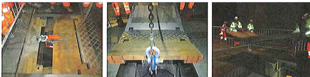
Removal of slide train
